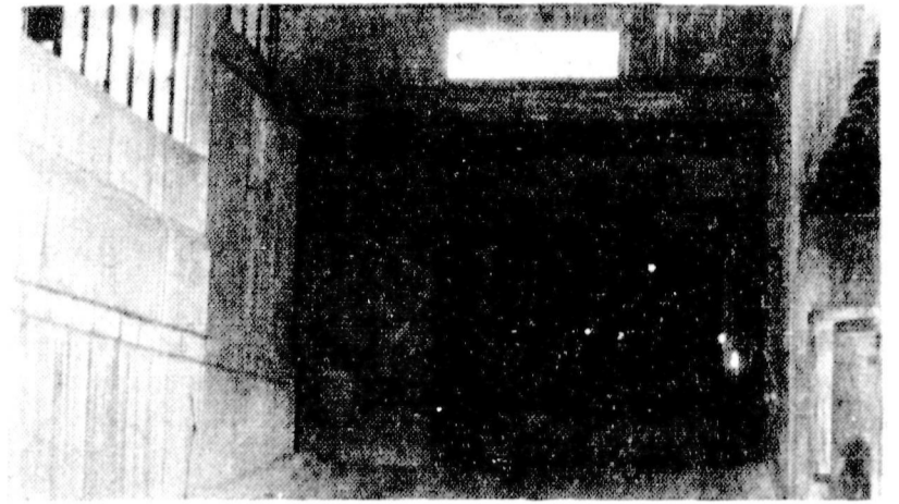
The danger tunnel next to the Earth Sciences Department
