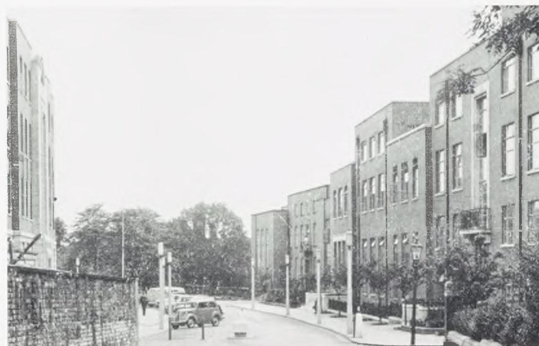
61b The north elevation of the Union and University House
