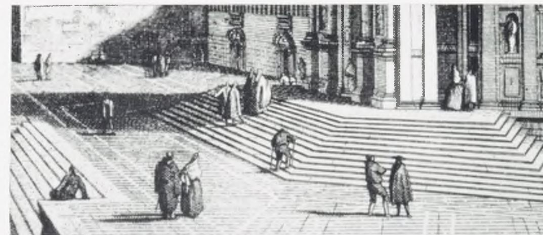
74a Terraces and steps
