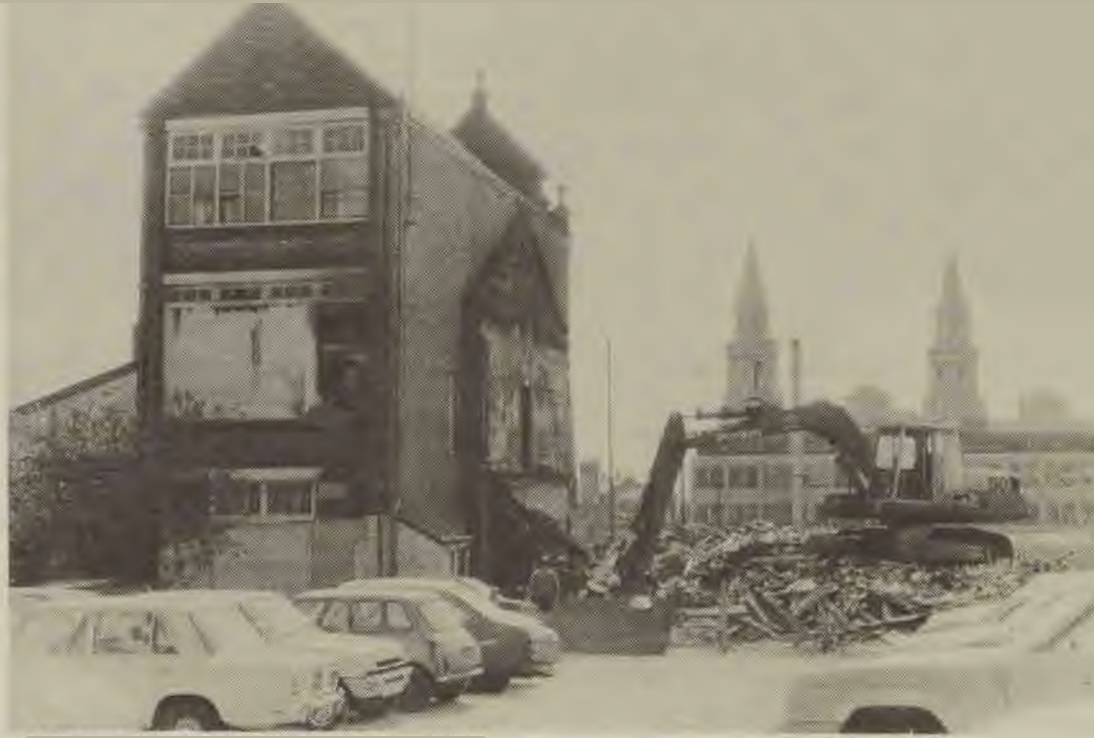
• The remains of Better Books are demolished.
