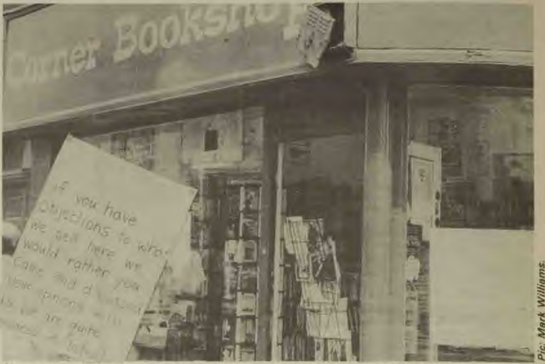
The damaged Corner Bookshop. The poster in the window is superimposed on the main photograph. Pic: Mark Williams.
