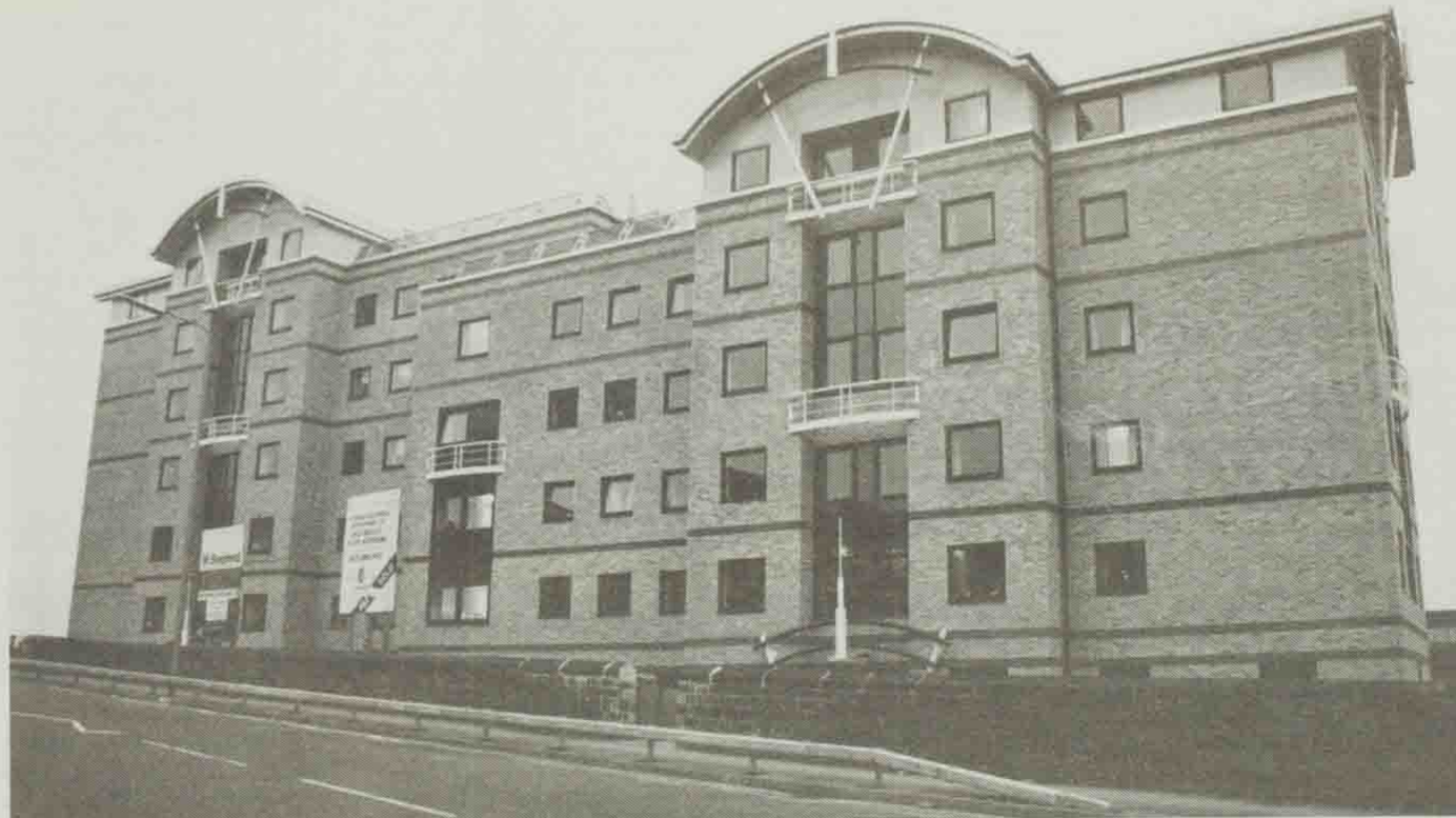
Sentinel Towers is plagued with problems and sky high rents were the last straw
