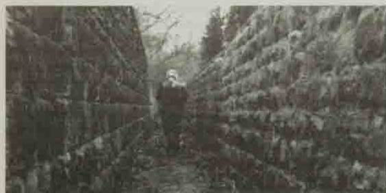
DANGERPOINT: The path next to Oxley Hall
