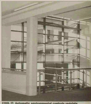
COOL IT: Automatic environmental controls regulate temperatures in TASC's new £5m state of the art building
