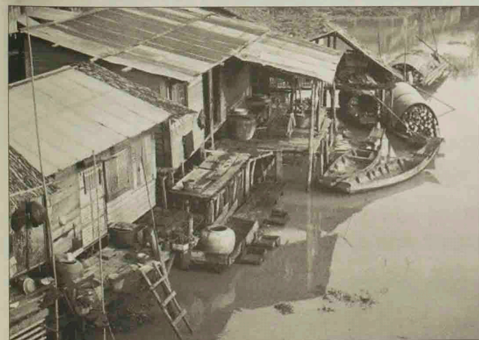
STILTED: Riverfront houses in rural Thailand built to withstand the seasonal monsoon floods
