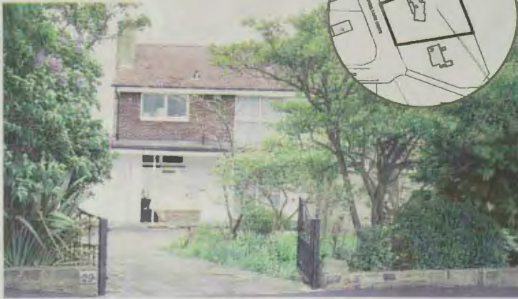
DEMOLITION JOB: Zaman's plans to tear down the house have been blocked by residents Photo: Laurie Whitwell
