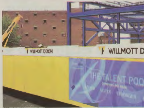
UNDER CONSTRUCTION: Work begins on the pool. Photo: Virginia Newman
