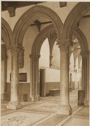
General Infirmary at Leeds, Entrance Hall.
