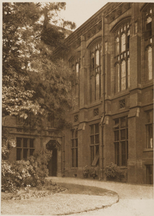
University of Leeds, Clothworkers' Court.
