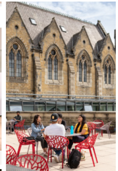
Rooftop terrace overlooking the Business School, western campus
