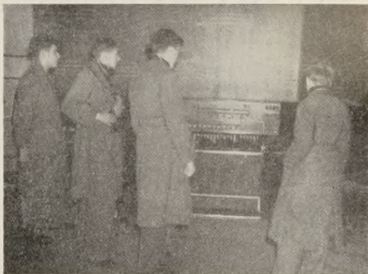
Railway Society inspect the re-signalling scheme at York
