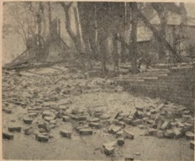
Gale damage near the Parkinson.
