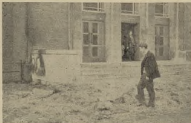
Scorched walls after Monday's fire.
