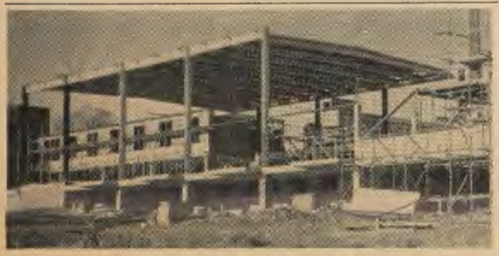
Structure of refectory now going up.
