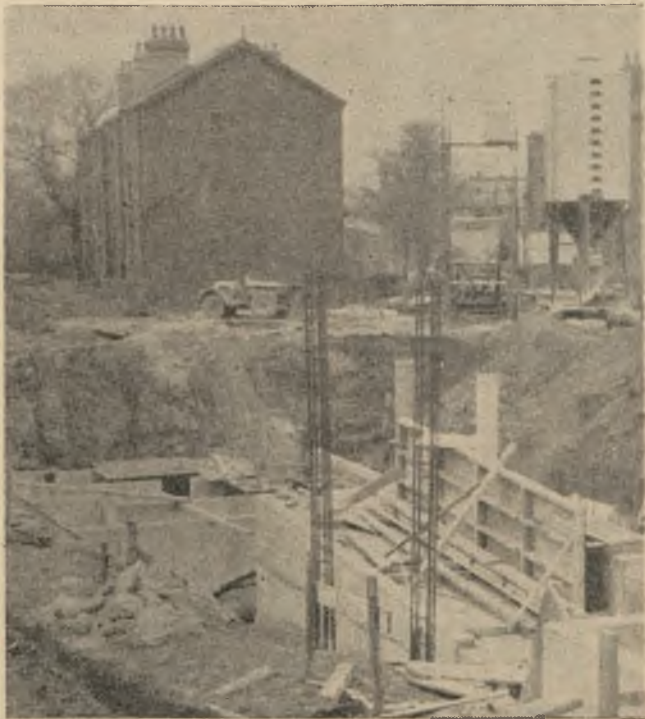
Work began last week on the Charles Morris Hall—the object of the Appeal. Picture shows the foundations.
