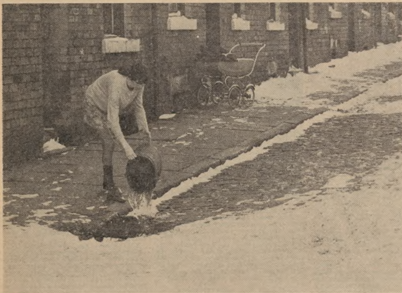
Kearney Street, Leeds 6. These houses have no sanitation and are due for demolition soon. But people still have to live in them. No drains, so this girl uses the gutter.
