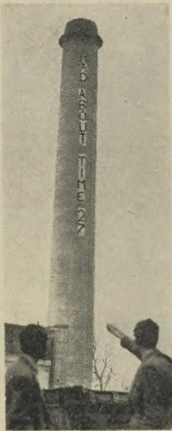
23.1.61. For their ball Engineers papered a 140ft. chimney as a stunt. For this they suspended someone in a bucket from the nearby crane.
