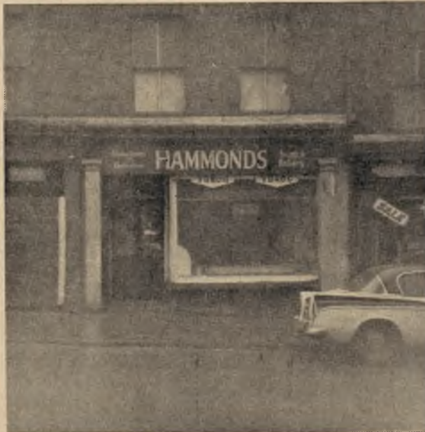
Hammond's — to be demolished soon.
