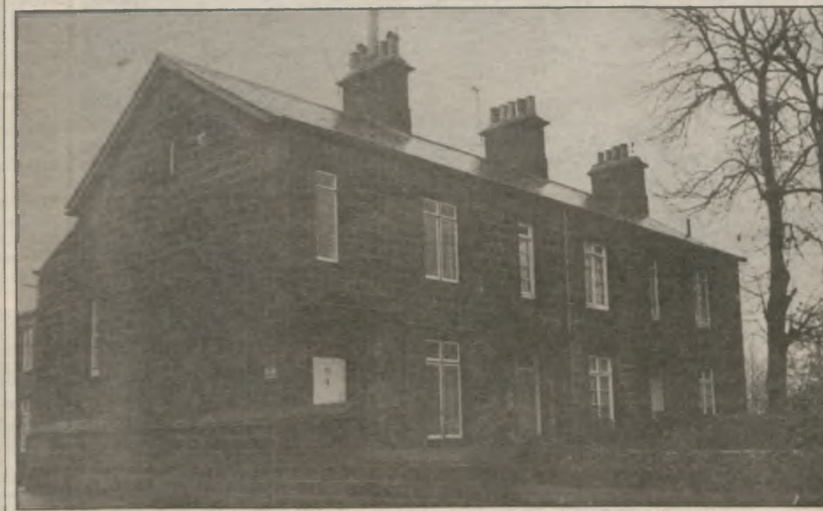
19th Century Cottages • Headingley
