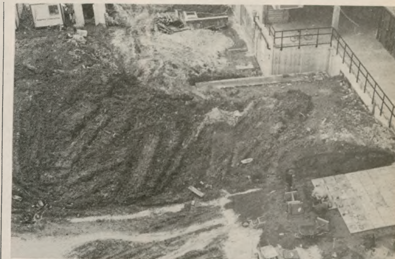
Landscaping in progress
